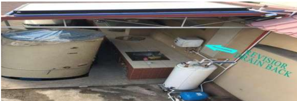
Fig.1. Modern solar gadgets use a self-draining technology called revisor drainage.
